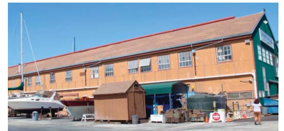
View of Building 12, East Facade
