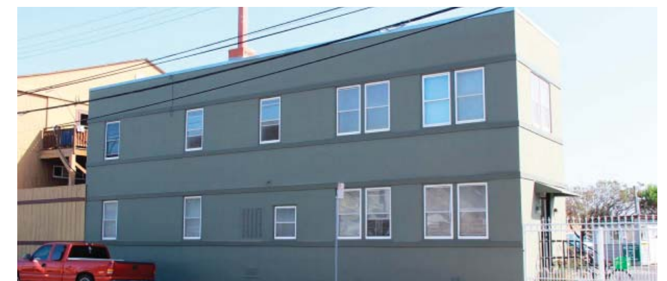
View of Building 27
