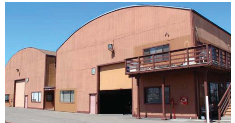
Buildings that are contributing to the “Alameda Marina Historic District”
