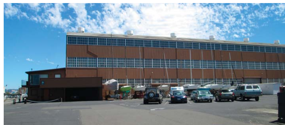
View of Building 19
