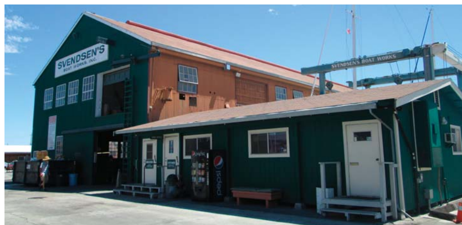
View of Building 12
