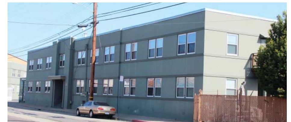
View of Building 16
