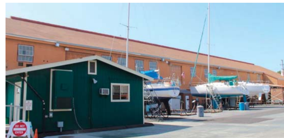
View of Building 12, West Facade
