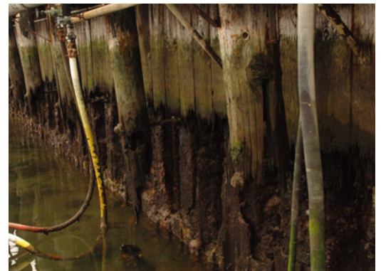
The existing shoreline is in need of rehabilitation and repair. Piles and shoreline the shoreline wall is rotting.
