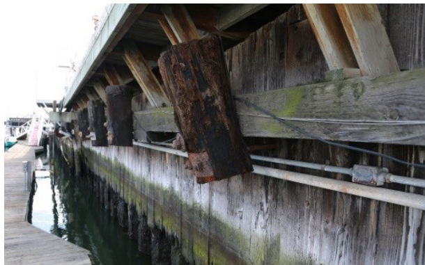
The existing shoreline is in need of rehabilitation and repair. Piles and shoreline the shoreline wall is rotting.
